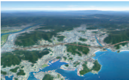
Manduk-Centrum Underground Expressway
